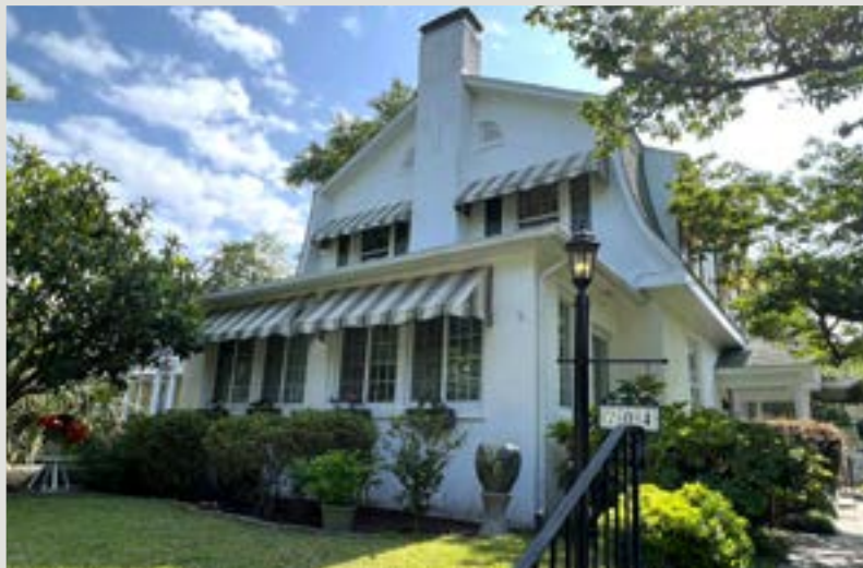
Dutch Colonial Revival House 204 North 15th Street
