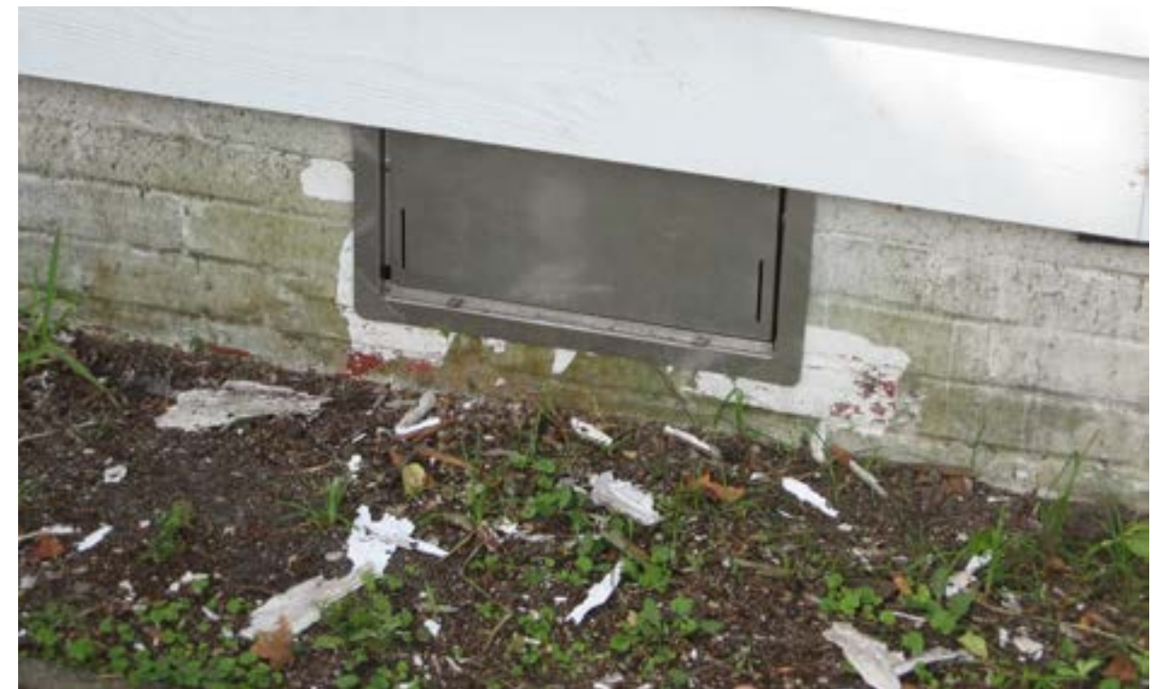
YES: Example of an appropriate metal vent in a low elevation foundation.
