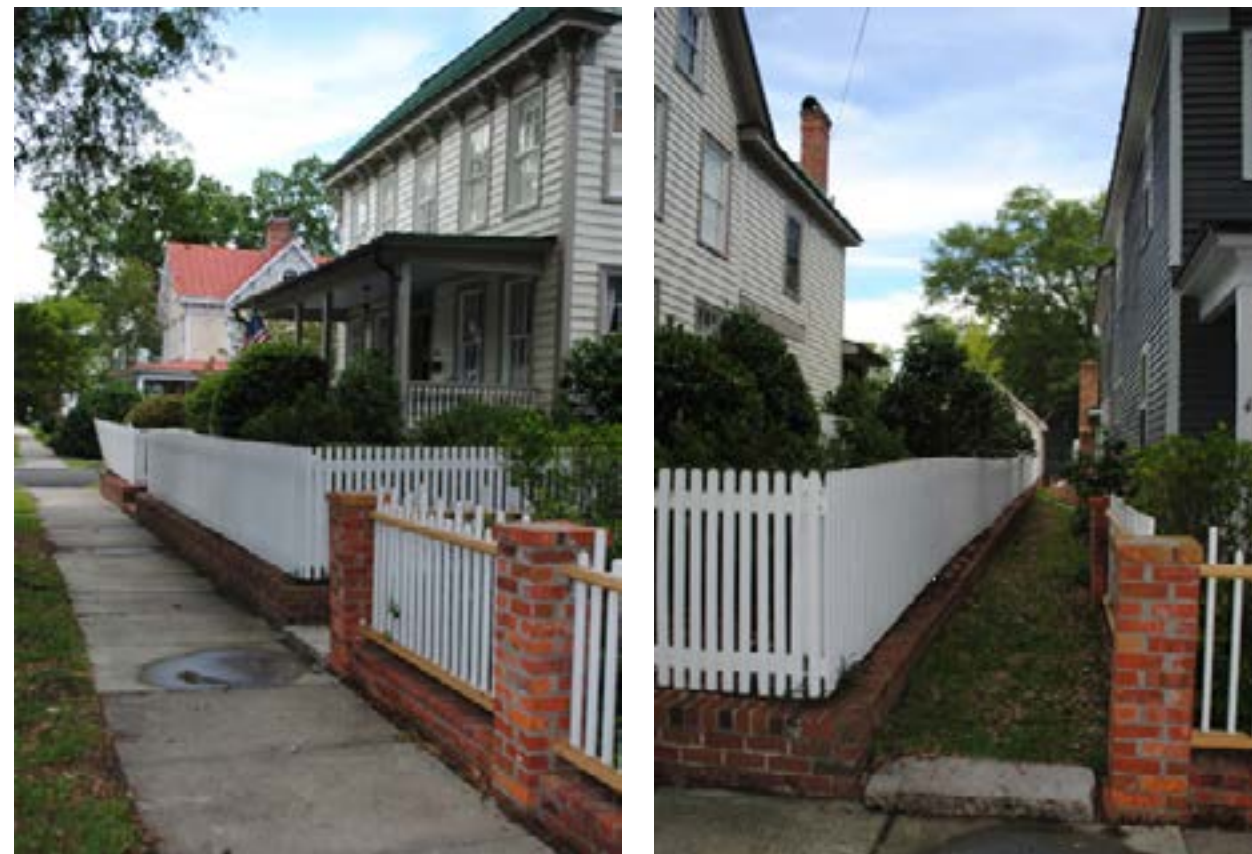
Low retaining walls and period fencing are used to screen the foundation of these low elevation increase projects.
