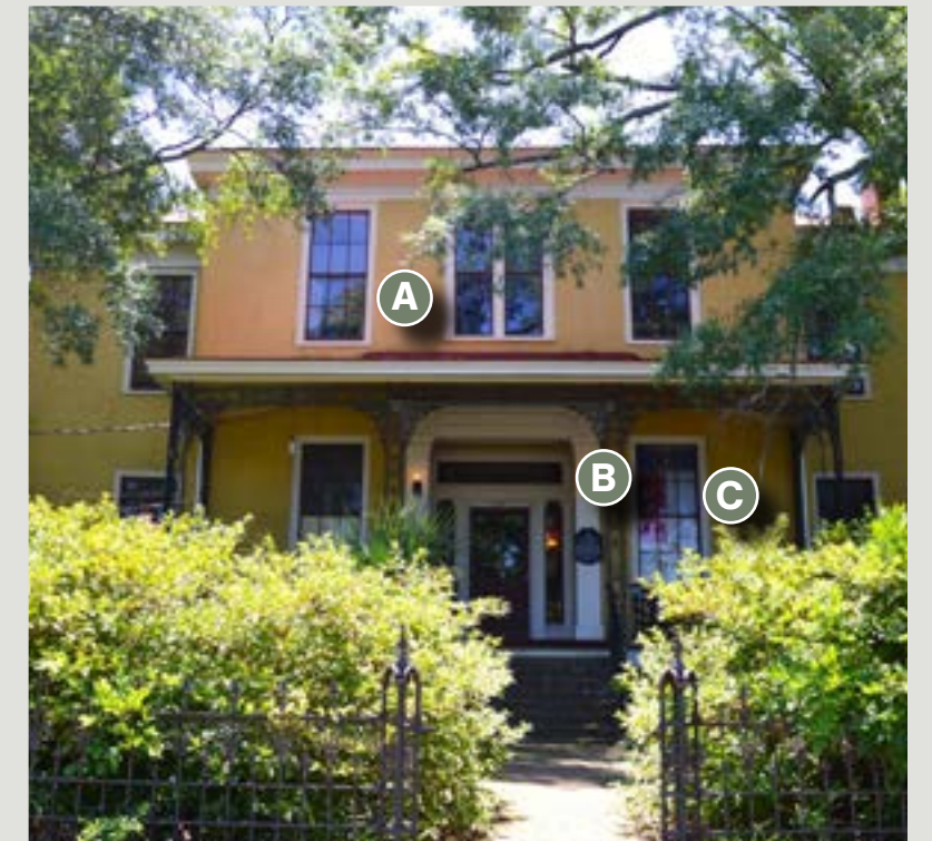
Federal House c. 1819 314 Grace Street
