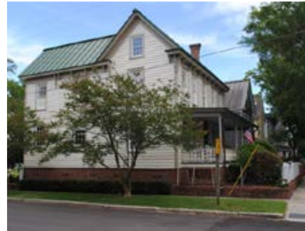
The screening of this low elevation increase project includes a retaining wall and landscaping to mitigate the increased height of the foundation.
