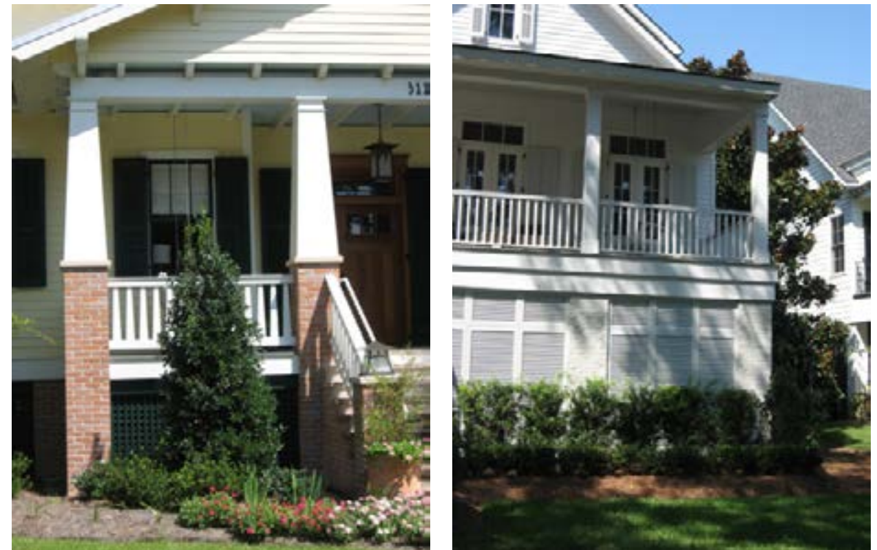
The porch columns and piers are in appropriate alignment in these photos of building elevations (above) and high increase building elevation (below).
