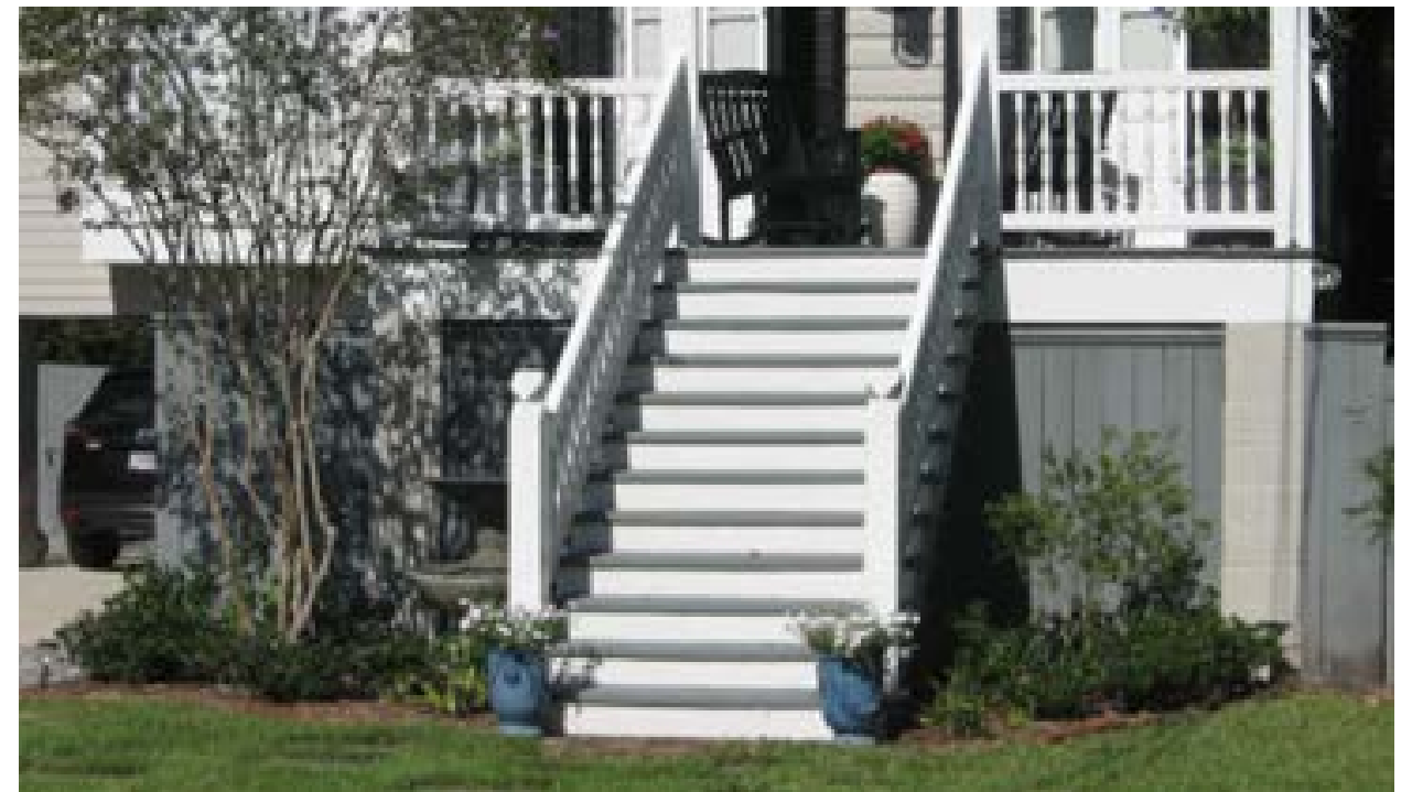
The wood stair complements the dwelling's style and design.
