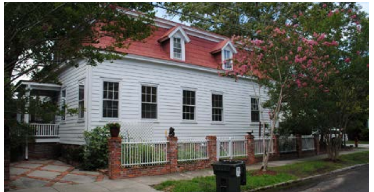
Above and below is an example of an appropriately sized retaining wall and period fence to screen the low elevation increase of this dwelling.
