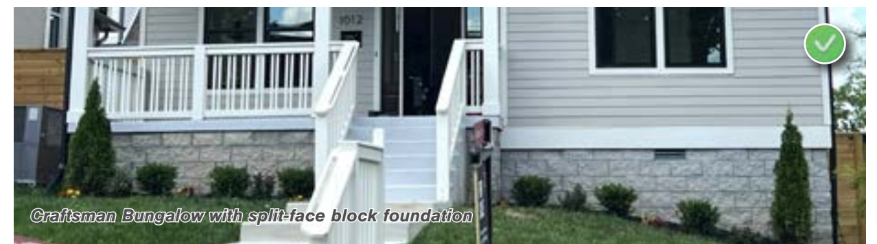
Examples of New Residential Buildings from other communities Source: The Walker Collaborative
