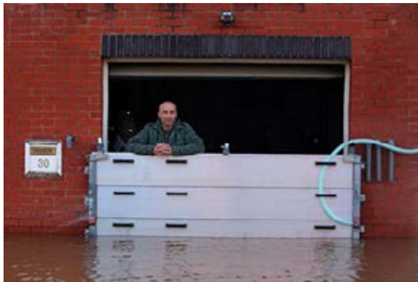
Floodproofing for commercial buildings can include the temporary addition of flood shields on doorways.
