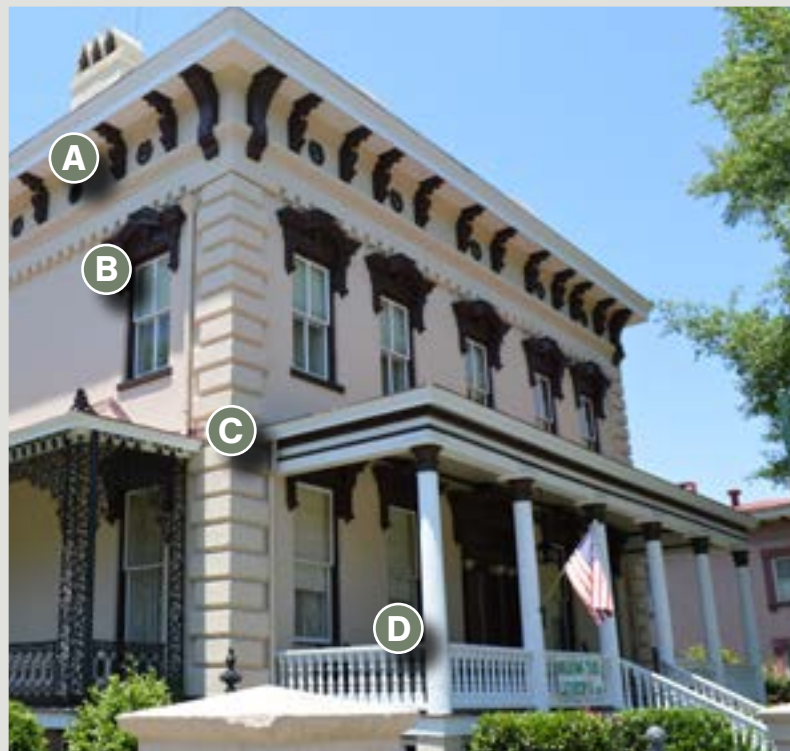
Italianate House c. 1852 126 South 3rd Street
