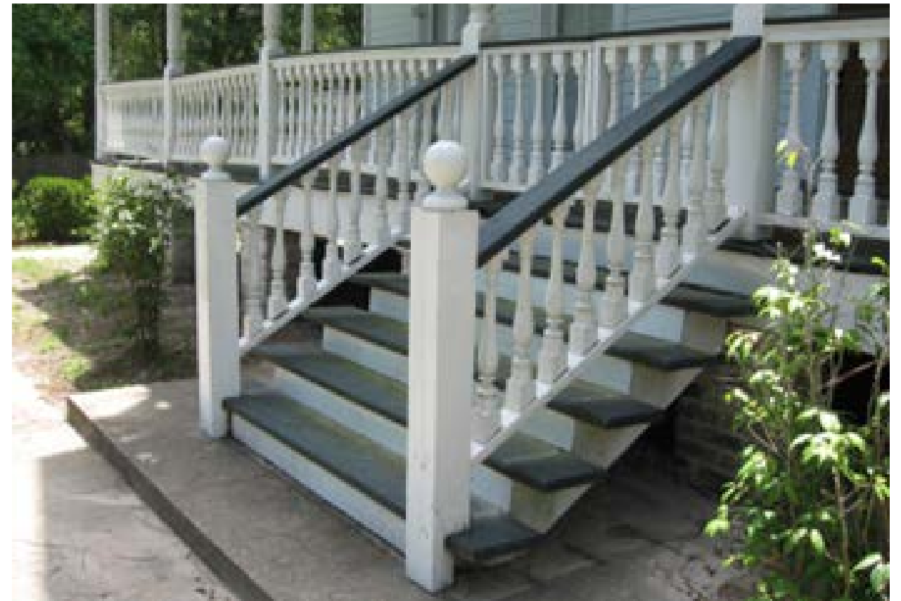
Rebuilt stairs should match the dwelling's original porch design and detailing.
