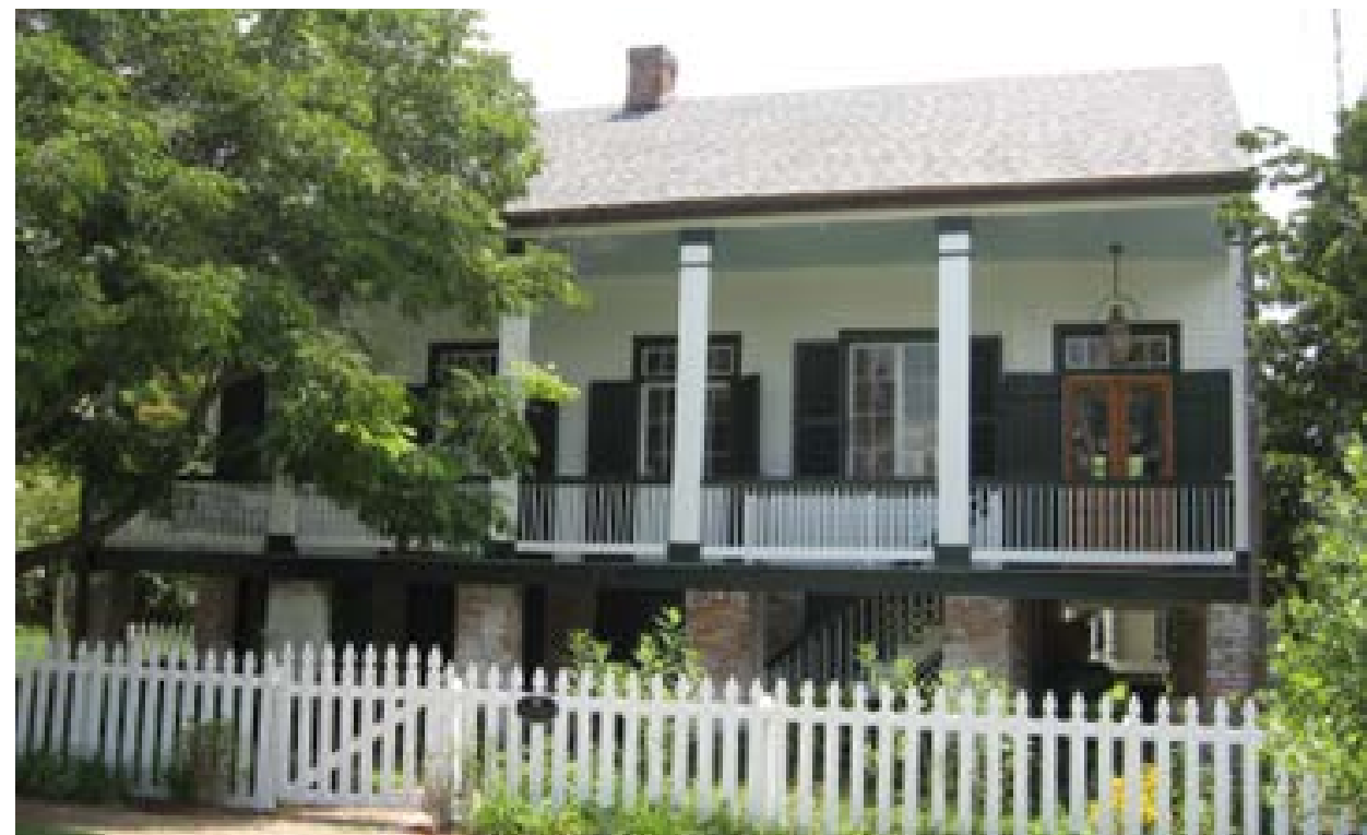
When elevating a dwelling a preferred option for an interior chimney is to retain the chimney and elevate it with the dwelling.
