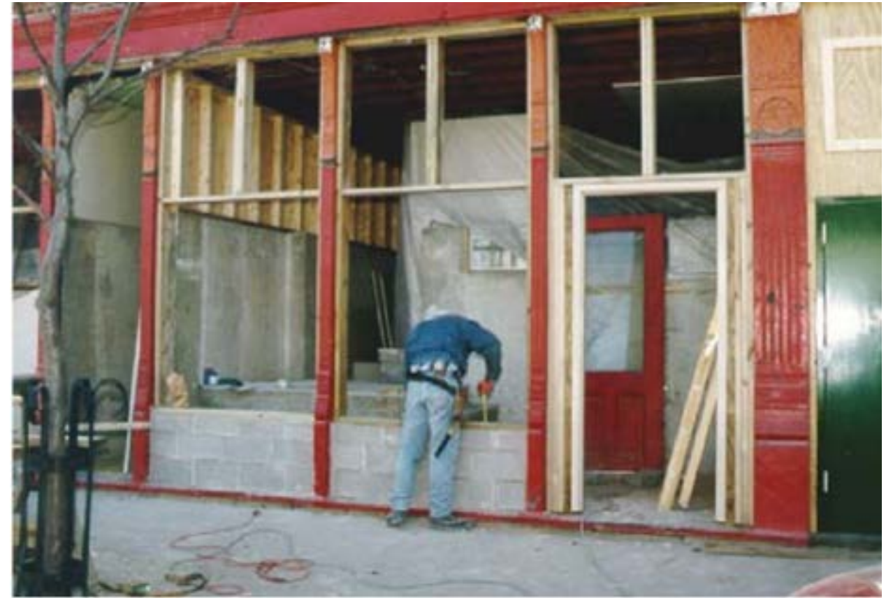
A strategy for floodproofing commercial buildings is to harden the storefront and raise the interior first floor level. In this approach the frame storefront bulkheads are replaced with concrete and a parged surface.
