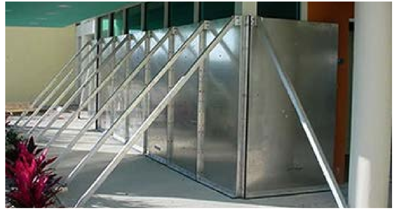
Temporary flood panels are now widely available to protect downtown commercial buildings. When high water events are anticipated these can be erected to minimize flood damage.
