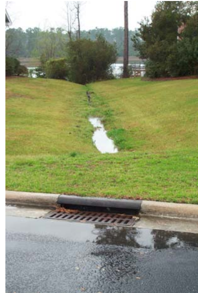
Grassed swale concentrating runoff into the riparian buffer from a residential area in the vicinity of Kestral Dr. Estuary pictured in background.
