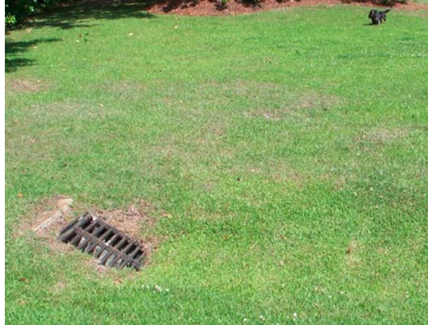
Waste generated from the dog pictured in the upper right-hand corner can enter the stormwater drainage system (and ultimately shellfishing waters) via this yard inlet.
