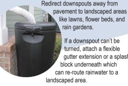
If a downspout can't be turned, attach a flexible gutter extension or a splash block underneath which can re-route rainwater to a landscaped area.
