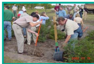
Workshop participants install a bioretention area in the Stormwater Demonstration Site at Anne McCrary Park.
