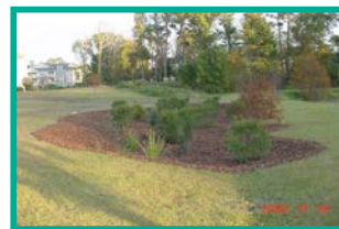
Workshop participants install a bioretention area in the Stormwater Demonstration Site at Anne McCrary Park.
