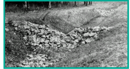
Check dams are barriers within a swale that are used to slow the speed of runoff and minimize erosion.
