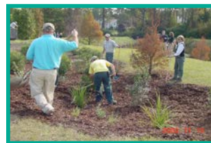
Workshop participants install a bioretention area in the Stormwater Demonstration Site at Anne McCrary Park.
