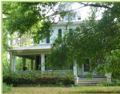
Fenley-Starnes House (3617 Wrightsville Avenue)
