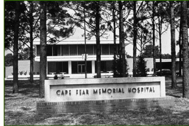
Cape Fear Memorial Hospital on Wrightsville Avenue east of Hawthorne Drive, courtesy of New Hanover County Public Library.
