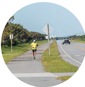
Highway 12 Sidepath Ocracoke Island, NC
