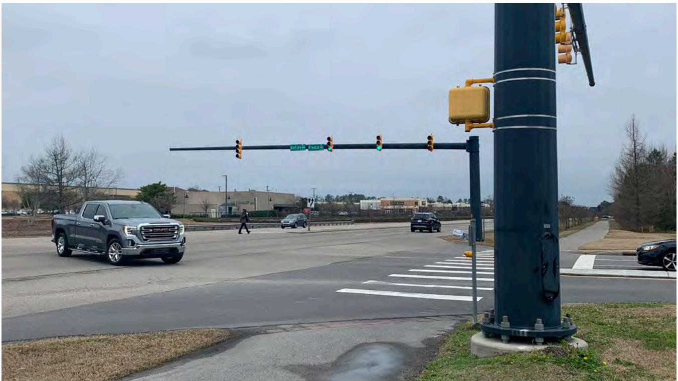
Sidewalk runs along Military Cutoff Road, but crossings of the major road are not provided at several intersections.
