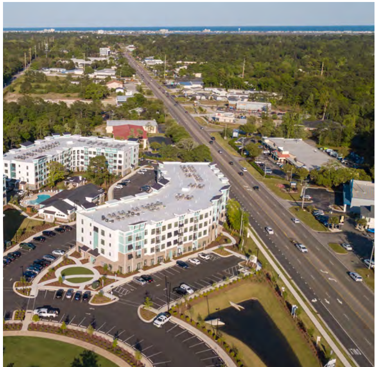
A new residential development including sidewalks and crossing improvements along Oleander Drive. Photo: Hawthorne Residential Partners
