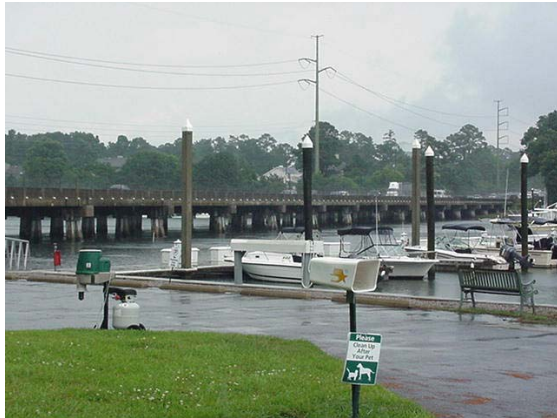
Image 9: Bradley Creek Bridge
