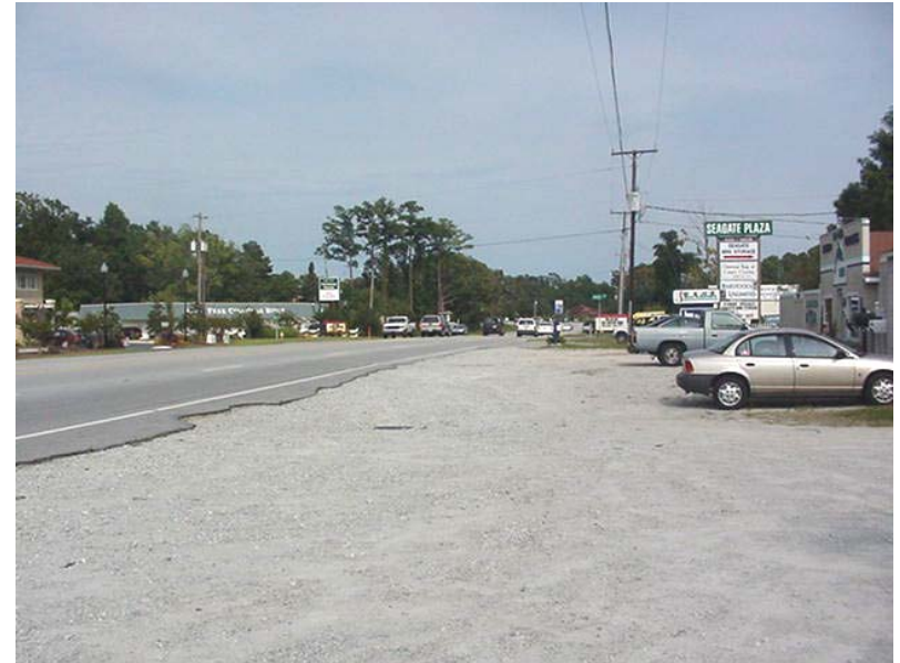
Image AD.2: A dilapidated portion of roadway with a lack of sidewalks, landscaping and trees.
