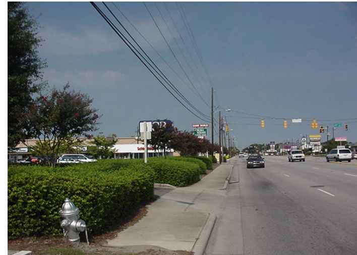
Image AB.3: View west toward 39 th Street. Sidewalks are directly adjacent to the roadway. Landscaping is moderate, with some trees. Power lines dominate the view.
