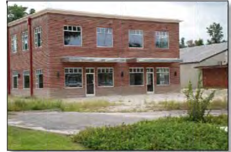
New development along Market Street
