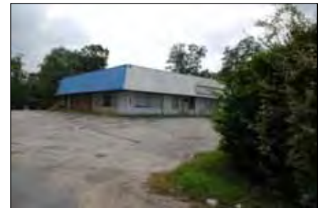
Dilapidated business along Market Street
