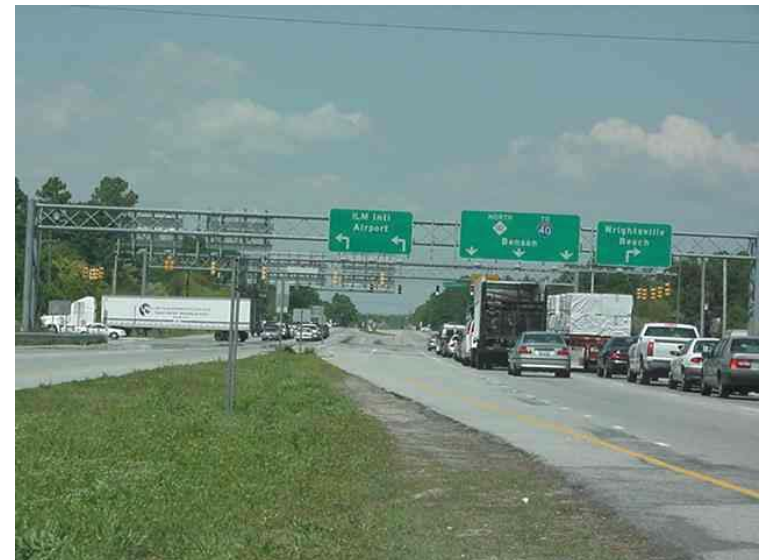
Image AA.2: Martin Luther King Jr. Parkway and College Road intersection
