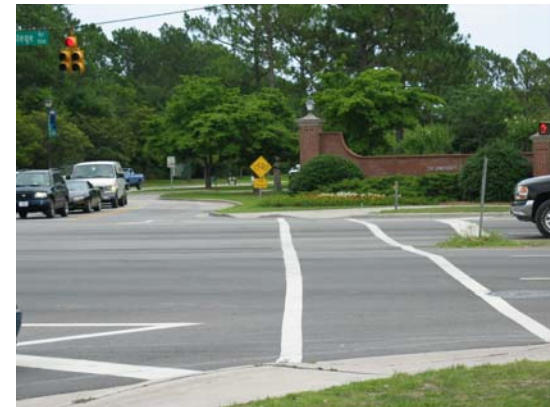
Image 13: Existing crosswalk at the Randall Parkway intersection
