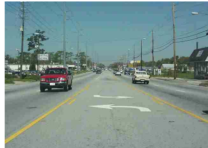
Image AB.2 This view south near Shipyard Boulevard illustrates the unprotected center two-way turning lane and the prominence of utility poles and lines.
