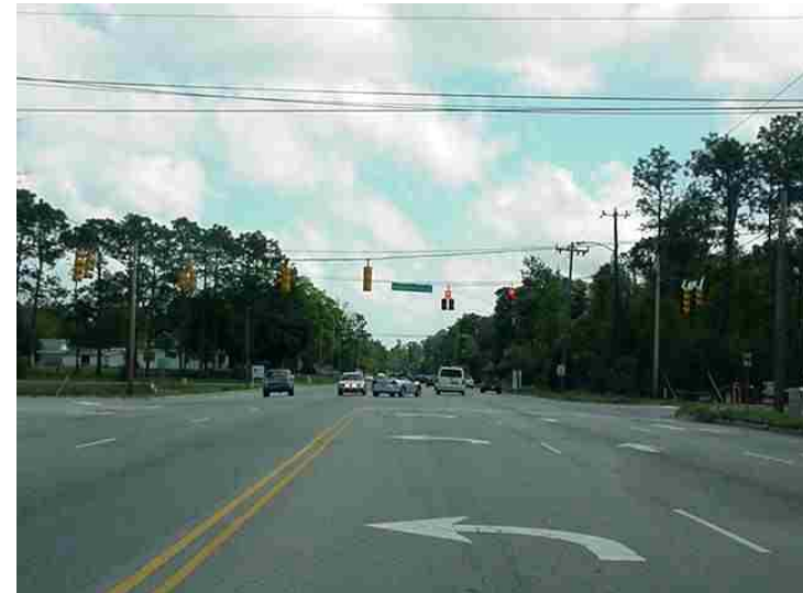
Image AD.2 Independence Boulevard intersection with left-turning lane.
