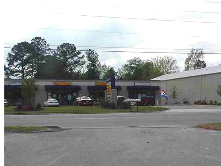
Image AC.1 Example of common strip style development with parking next to roadway and minimal landscaping.
