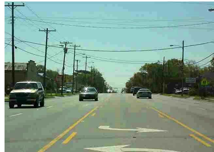
Image AA.2: View south toward Southern Boulevard. shows the unprotected center two-way turning lane and the prominence of utility poles and lines.
