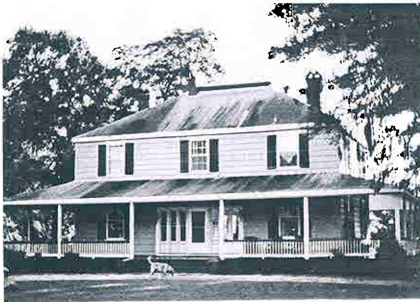
- The Latimer House has an unusually deep, one story porch wrapping around all four sides -photo courtesy of Mr. and Mrs. James C. Fox, Jr.
