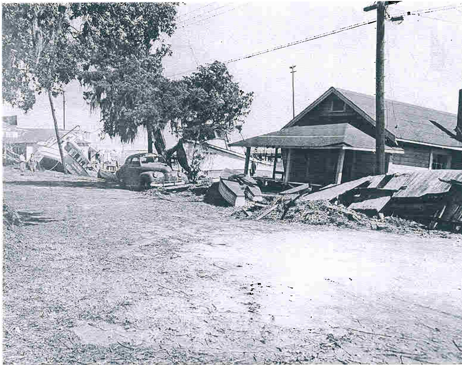
In 1954, Hurricane Hazel caused extensive damage along Airlie Road -photo courtesy of Maybert Lance.
